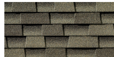
Roof Shingles: Weathered Wood
